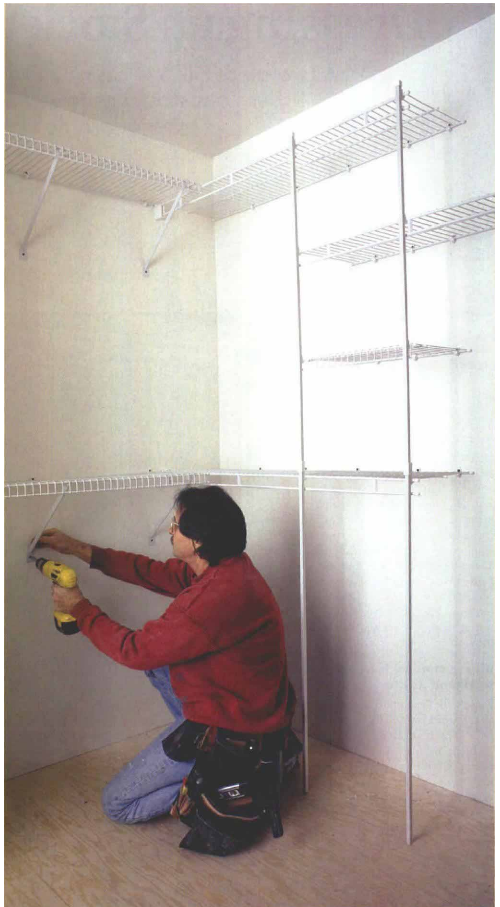
Angle braces support the shelves. Braces that snap into the wire shelving and screw to the wall reinforce long spans and support the shelves' ends where they meet in a corner.
