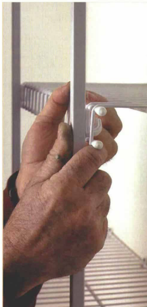
Clips on the poles hold the fronts of the shelves. While clipped to the wall, the shelves pivot up and snap to the poles.
